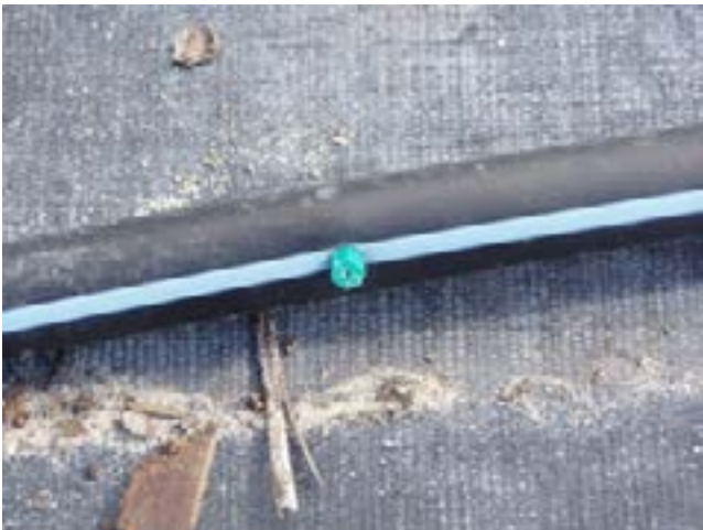
Figure 7-6 A microspray emitter with no moving part
