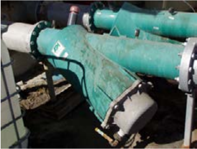
Figure 7-28 A large-diameter, steel, in-line screen filter
