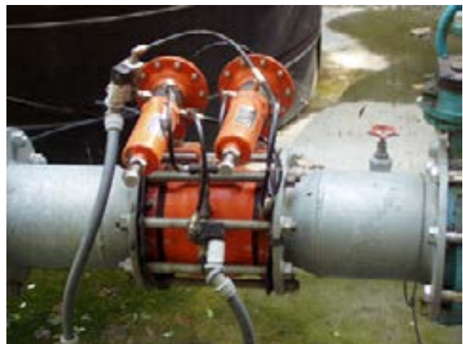
Figure 7-40 Solenoid controlled, pressure regulating valve
