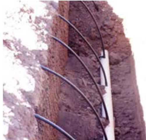
Figure 7-3 Permanent SDI hose and manifold used for field and vegetable crops
