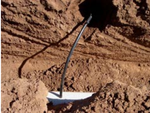
Figure 7-52 Permanent SDI manifold used for field and vegetable crops. Similar manifolds can be used for tree and vine crops using different lateral spacings
