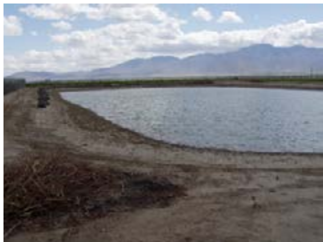
Figure 7–38 A well maintained settling basin
