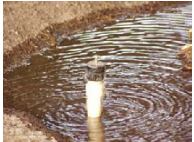
Figure 7-4 A bubbler discharging water into a small basin around the tree
