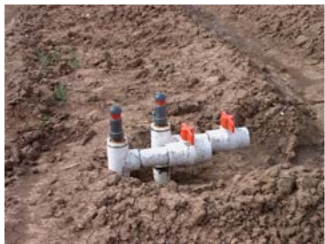
Figure 7–43 Automatic continuous acting air release valve
