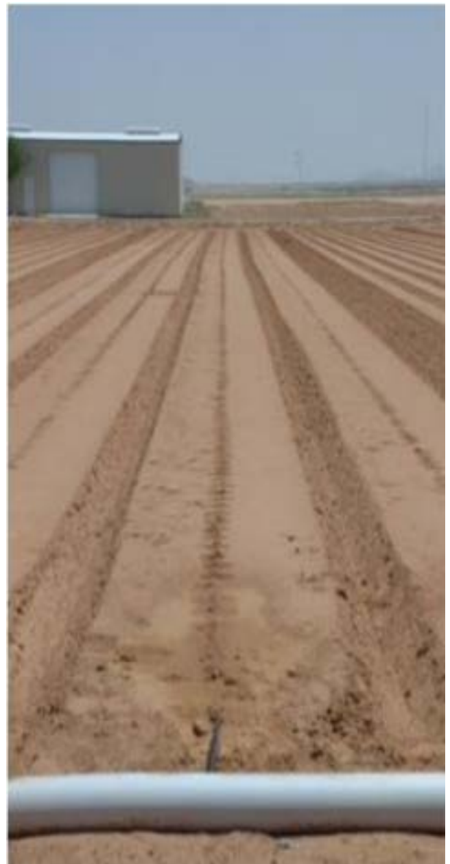
Figure 7-122 A 300-foot-long (94 m) LPS lateral and the connection to the polynet manifold
