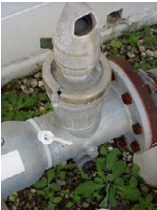
Figure 7–42 Air/vacuum relief valve
