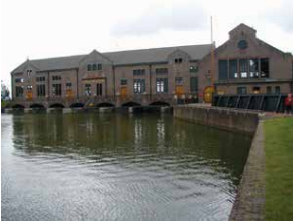
Figure 17.12. The Wouda pumping station was built to drain large areas in Friesland, Netherlands, and is the largest steam pumping station ever built. It is now on the World Heritage List.
