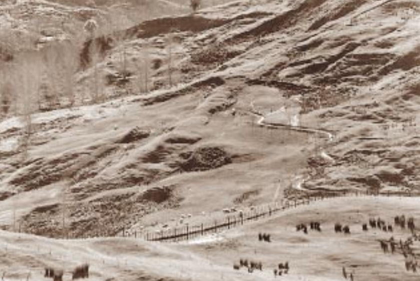
Surface recontouring of an earthflow north of Gisborne. The areas of recontoured, smoothed and cultivated land contrasts strongly with the areas of untreated earthflow. A graded bank removes water from an area of springs to stable land for safe disposal. Photo: Don Miller.
