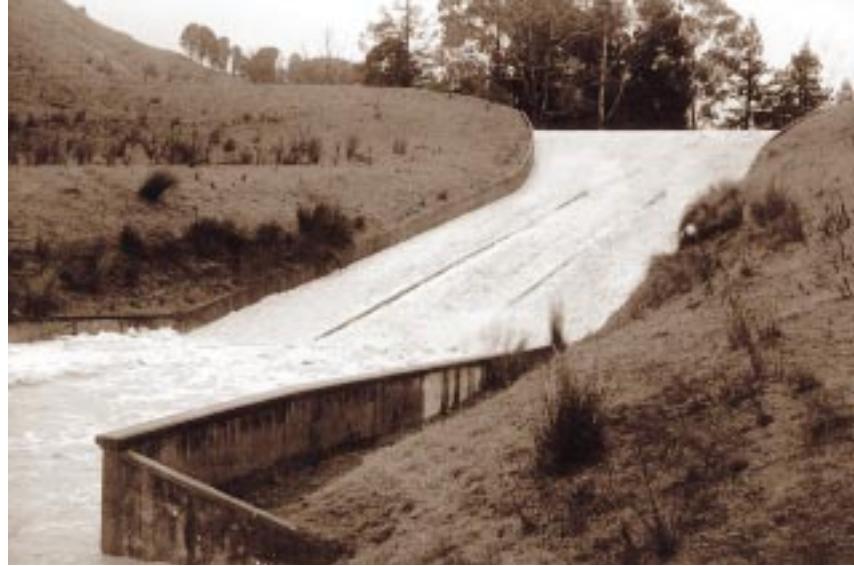
Concrete drop structure – spillway over dam.
