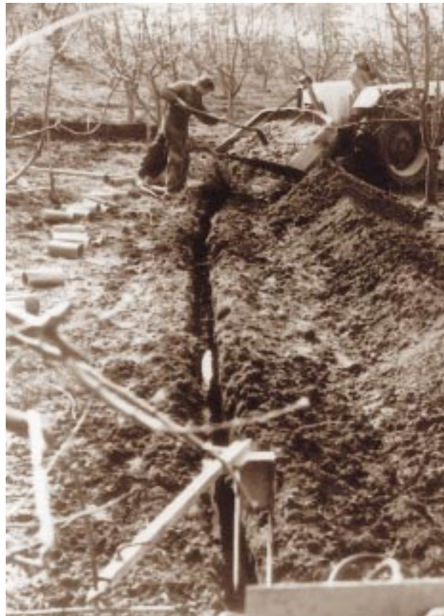
Installation of tile drains through orchard.
