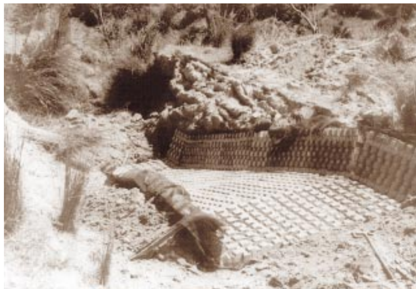
Geotextile interlocking concrete blocks.
