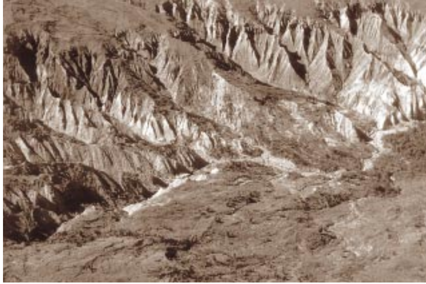
V shaped gullies on crushed argillite country.
