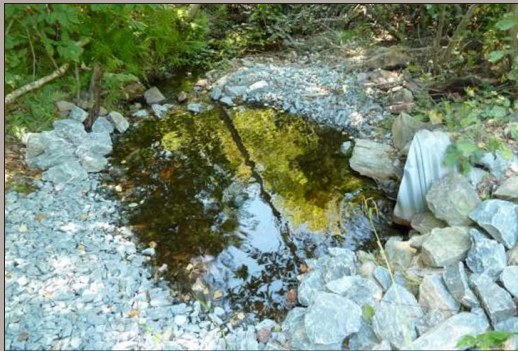
I-6: Use of flow dissipaters to minimize erosion at discharge point.
