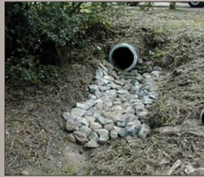
I-6: Use of flow dissipaters to minimize erosion at discharge point.
