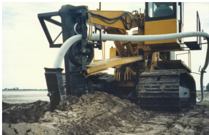
Figure 20. Laying corrugated drainage in citrus bed with plough-type drain installation machine.
