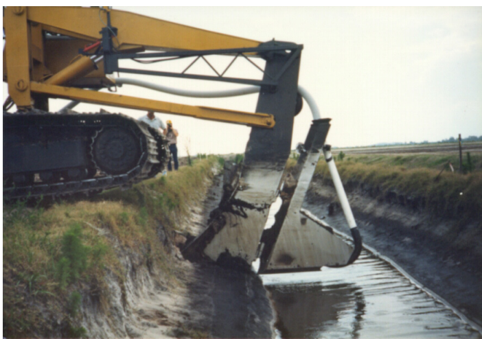
Figure 19. Installing 4-inch corrugated drain tubing with PVC pipe discharge.
