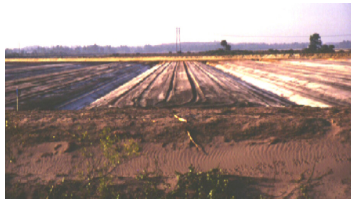
Figure 9. Double-row bed under construction.
