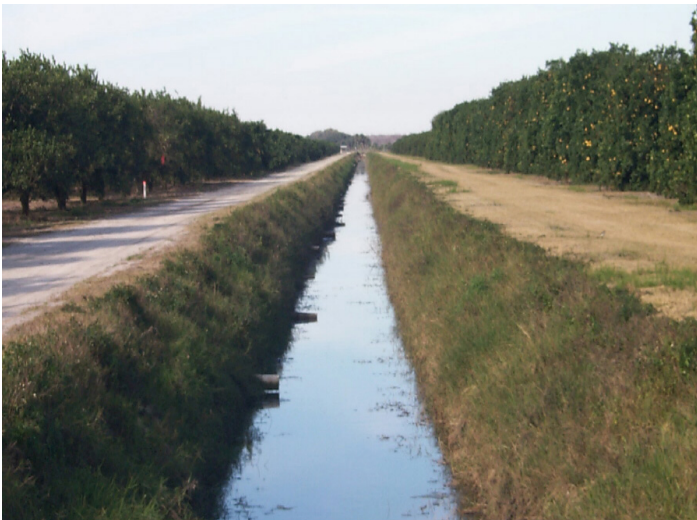
Figure 11. Lateral drainage ditch with water furrow outlet pipes discharging into ditch.
