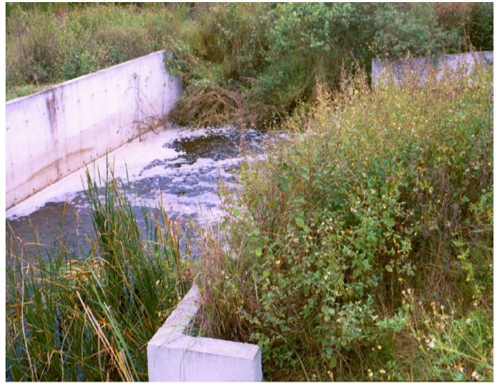
Figure 16. Erosion control structure on grove discharge canal.
