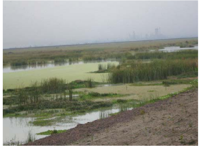
Figure 43. Constructed wetland for treatment of fly ash slurry
