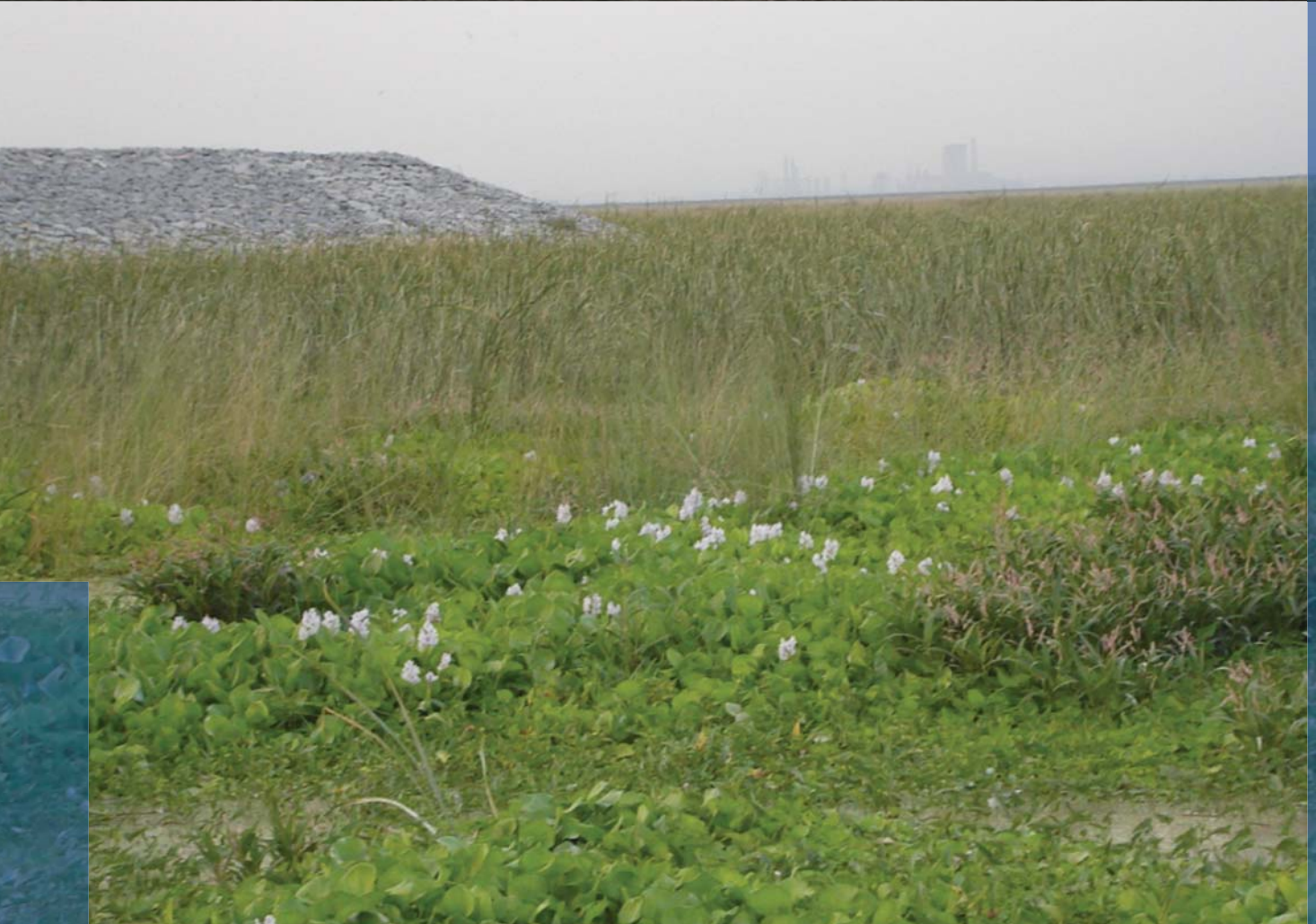
Constructed wetland at NALCO's Angul plant in Orissa with macrophytes for treatment of coal fly ash slurry released from captive power plant
