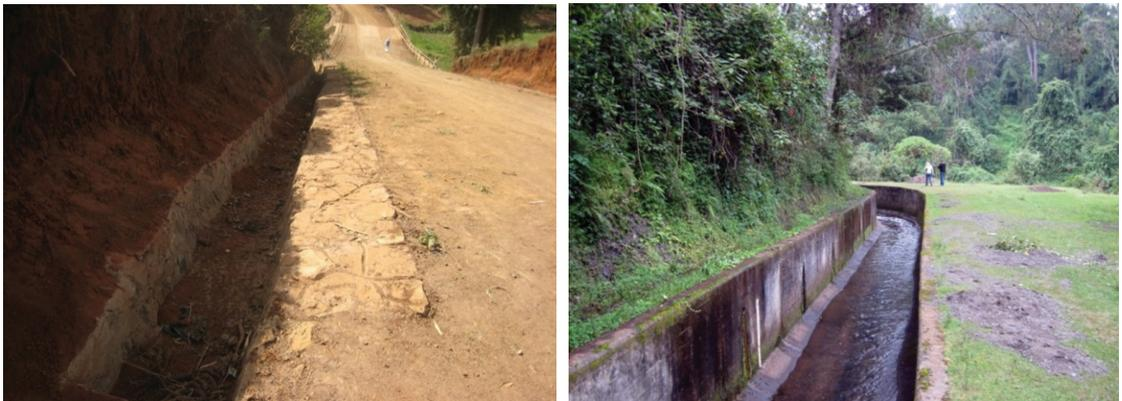
Figure 12-3: Concrete lined cut-off drains in Kapingazi, Embu Kenya.<sup>35</sup>
